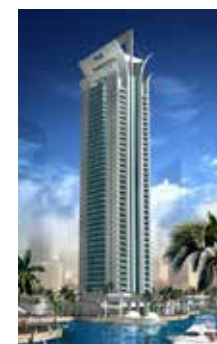
Jumeirah Lake Tower Dubai, UAE
